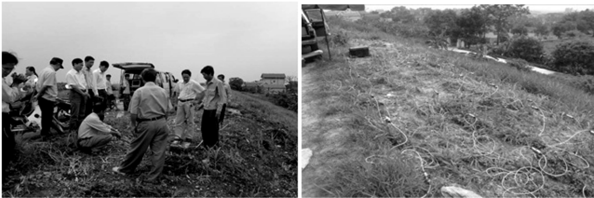
Fig. 5. Identifying the hollow caves by Ground penetrating radar and multi-electrode at K112+697 position of the Red River right dam.
