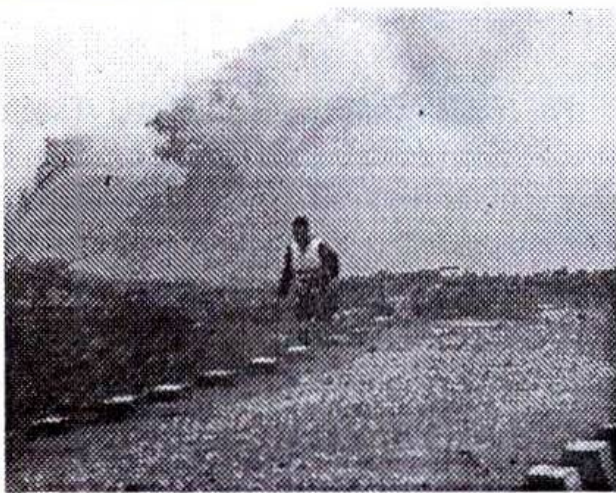
Photo 4. Sea dyke Do Son I during the storm No. 7, September 2005.
