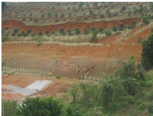
Figure 2. 2018 landslide in farming slope in the red mud basin No. 2 - Nhan Co alumina factory.
